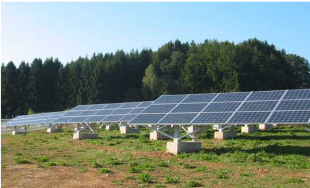
Photo Plate 4: Proposed Fixed Tilt Mounting Structure (Source: Conergy)
