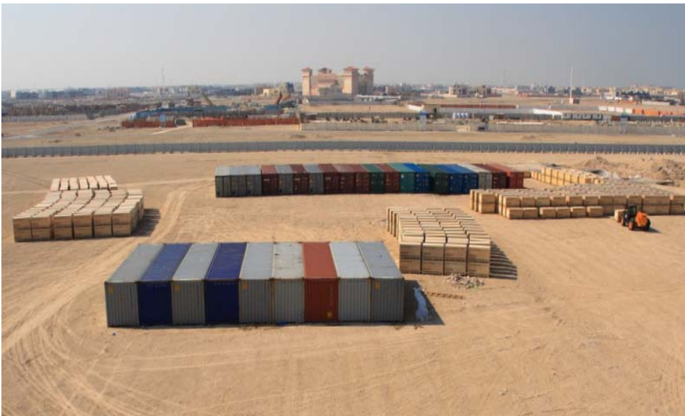
Photo Plate 10: Staging Area for a Solar Facility
